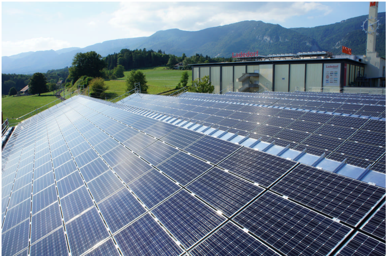
Figure 2: Finished roof surface
