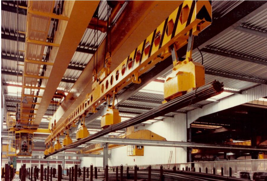
Figure 2: Taking a rebar bundle from between the uprights
