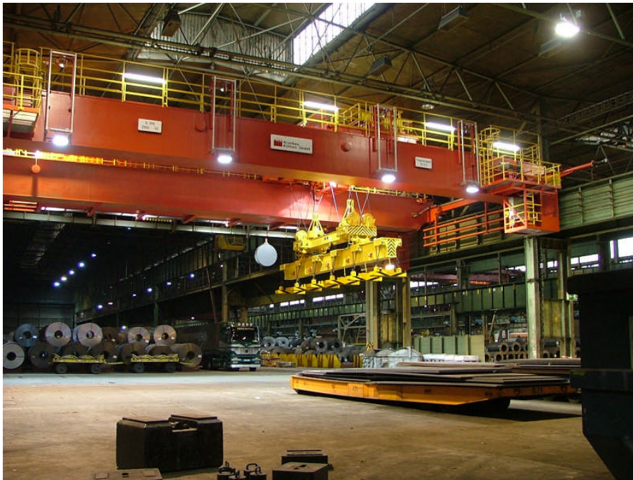
Figure 1: Magnet spreader beam in a steel mill
